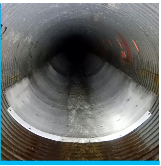
In 2019, Concrete Canvas® (CC8) was used for the rehabilitation of an existing 2,100mm diameter, structural plate corrugated steel pipe approximately 372m in length at the Mackinnon Ravine storm trunk near 149th street in Edmonton, AB. Existing deficiencies in the culvert storm trunk included high ovality deformation, invent corrosion and joint separation.
