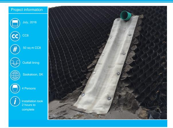
In July of 2016, 50 sq. m of Concrete Canvas 8mm (CC8) was used to line 8 outfalls on the side slope of a roadway in Saskatoon, SK, Canada. Each outfall was approximately 1m wide and 6 m long.
