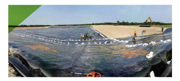
Geomembranes are used with rocks or earth to block fluid migration in man-made structures. They are manufactured in sheets ranging from 0.25 to 3.5 mm in thickness and are made of various synthetic materials such as EPDM (Ethylene Propylene Diene Monomer), Linear Low-Density Polyethylene (LLDPE), High-Density Polyethylene (HDPE), Polyvinyl Chloride (PVC), and Polypropylene (PP).
