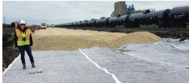
Post-installation showing TE-BXC30 soil reinforcement performance.
