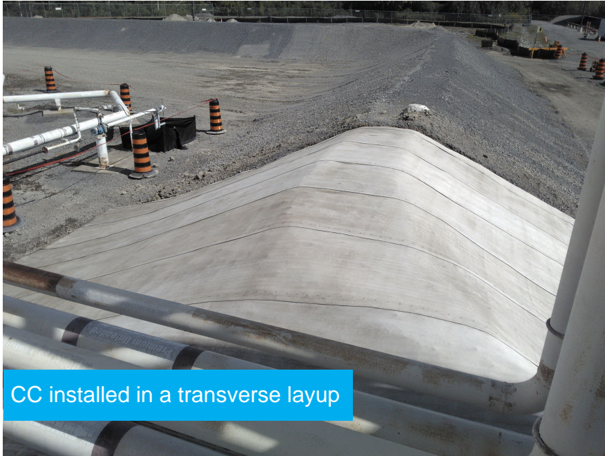
CC after HDPE liner installation
