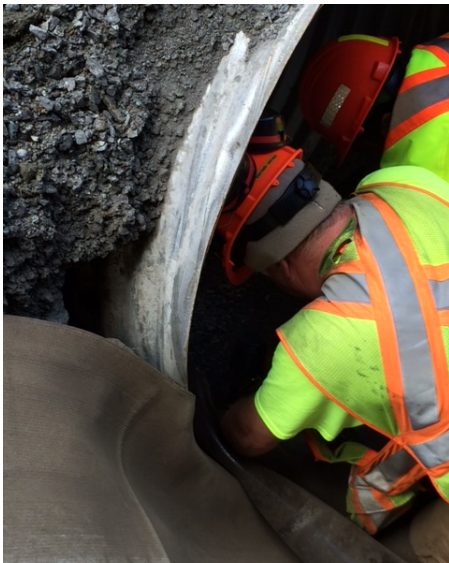
Fastening CC to inside of culvert
