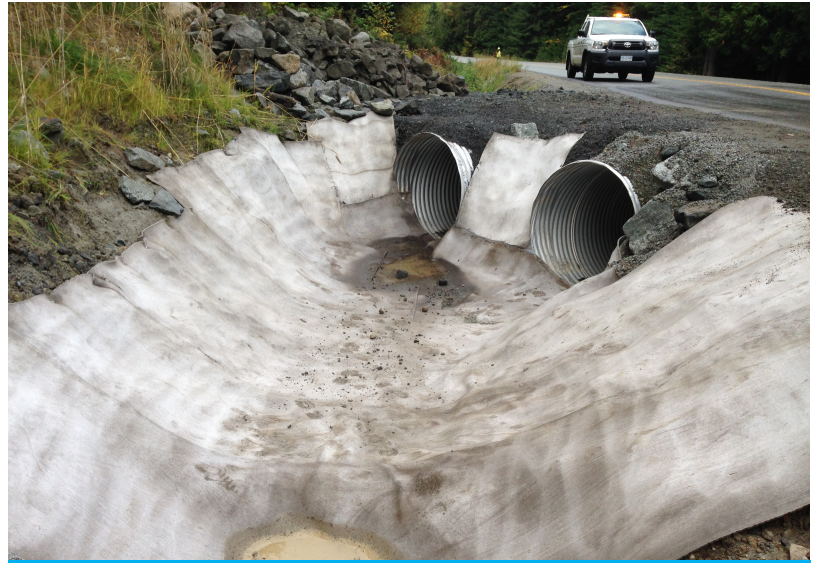
Completed CC installation
