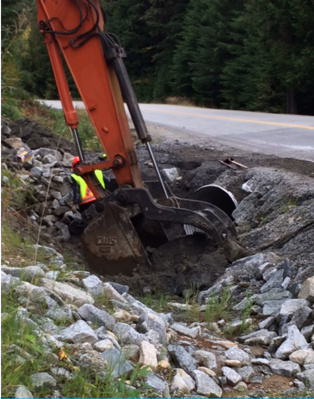
Site prep included regrading of the ditch profile
