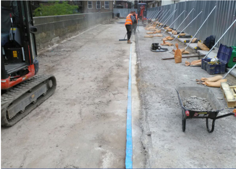
Completed section re-covered with CCH edge exposed for welding
