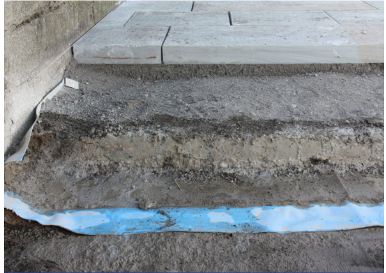
CCH layer underneath re-layed substrate and flagstones
