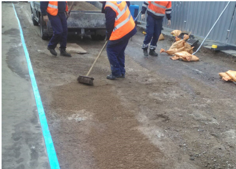
The substrate was flattened before installation
