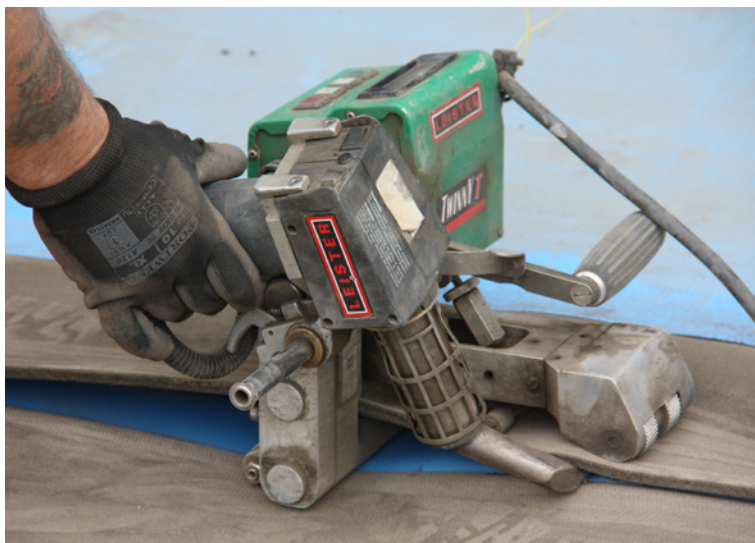
CCH joints were welded with Leister Twiny Ts and Triacs
