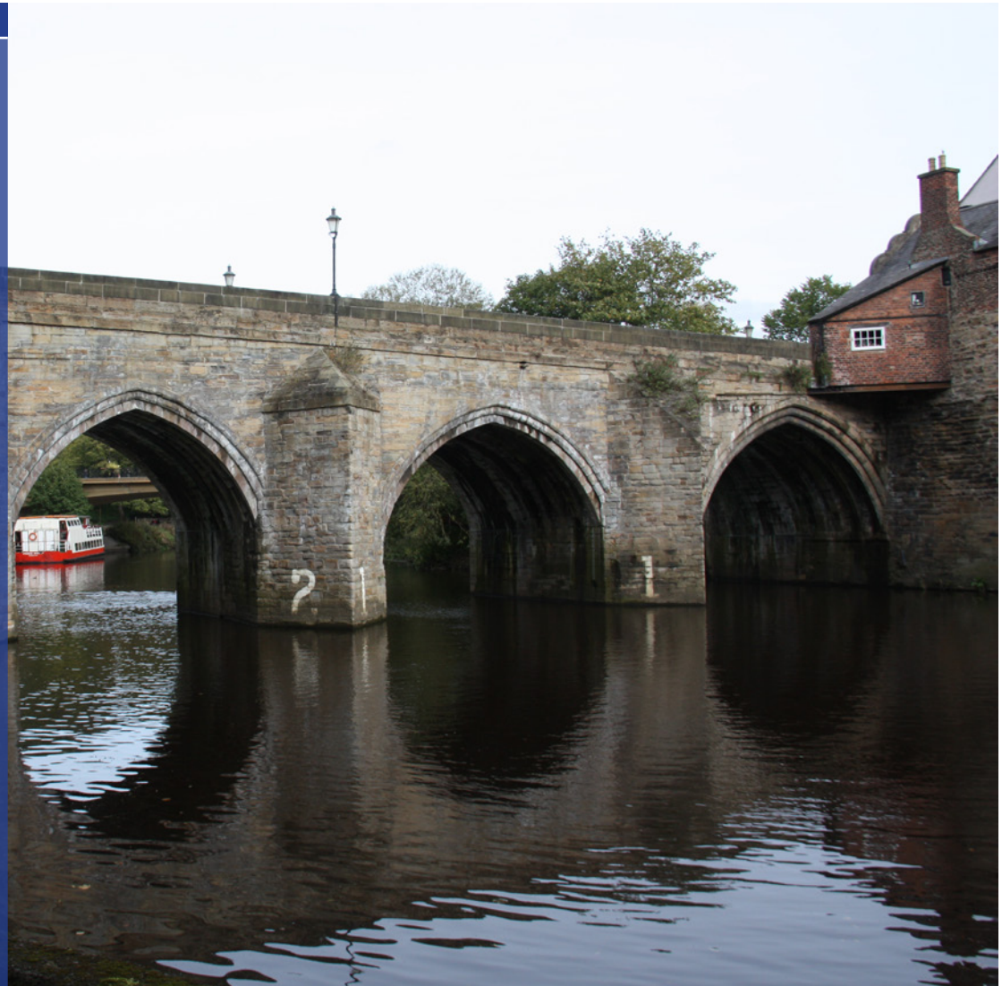
A view of the bridge from across the river
