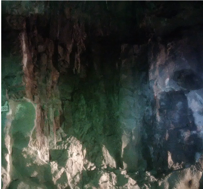
Walls all cleaned off of crumbling material
