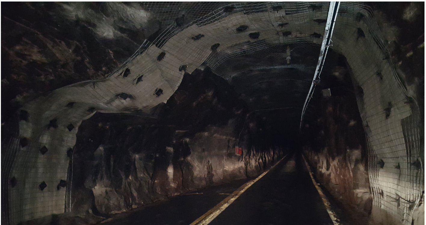
One of the four completed tunnel sections
