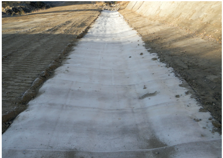
Completed channel trial installation
