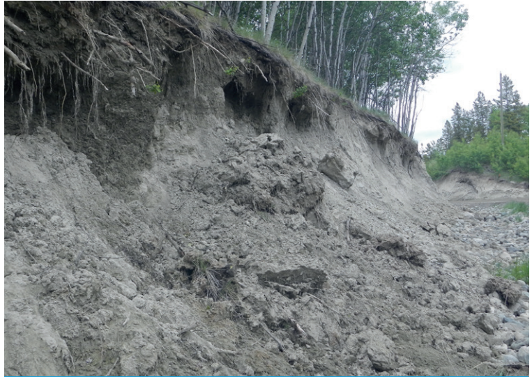
Sand-based substrate in the area was prone to erosion
