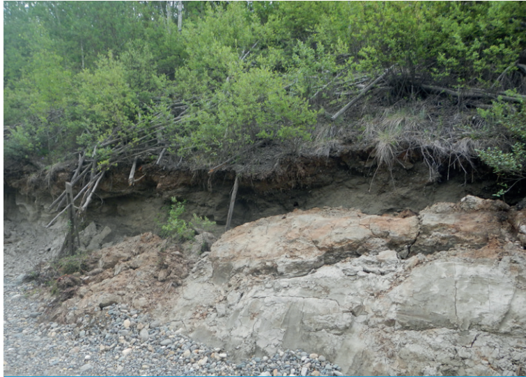
Condition of slope prior to installation
