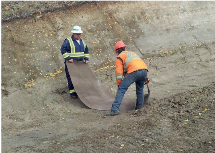
CC8 was cut to length and laid transversely
