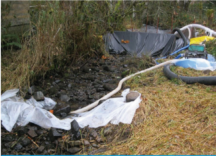
Isolating with cofferdams
