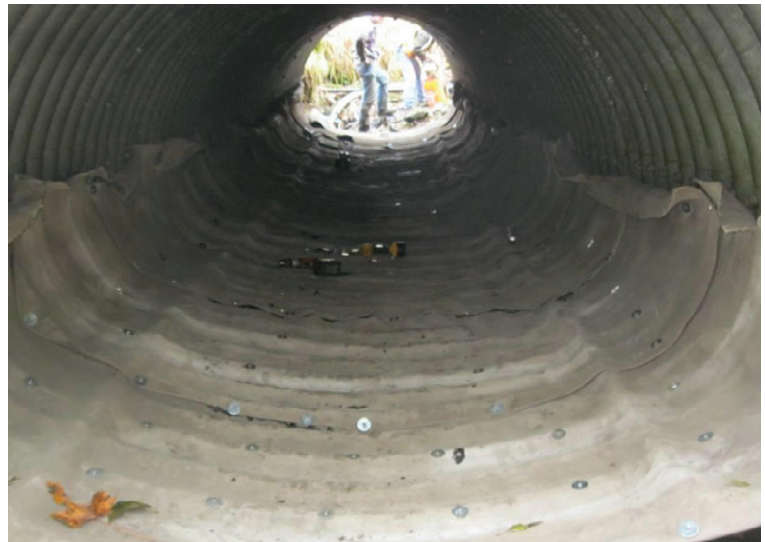
CC post-installation, prior to trimming and sealing of edges
