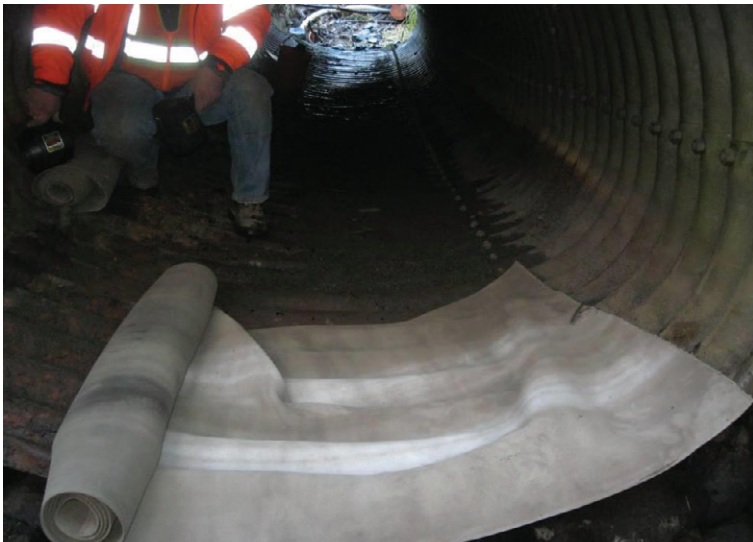
CC laid transversely across culvert floor
