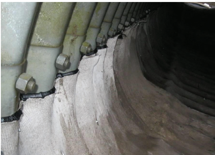
Tar used to seal material edges
