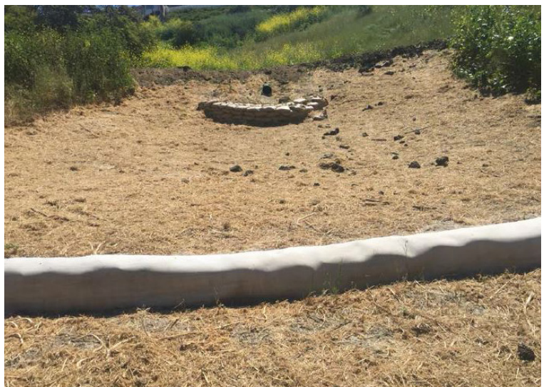
Completed baffling section
