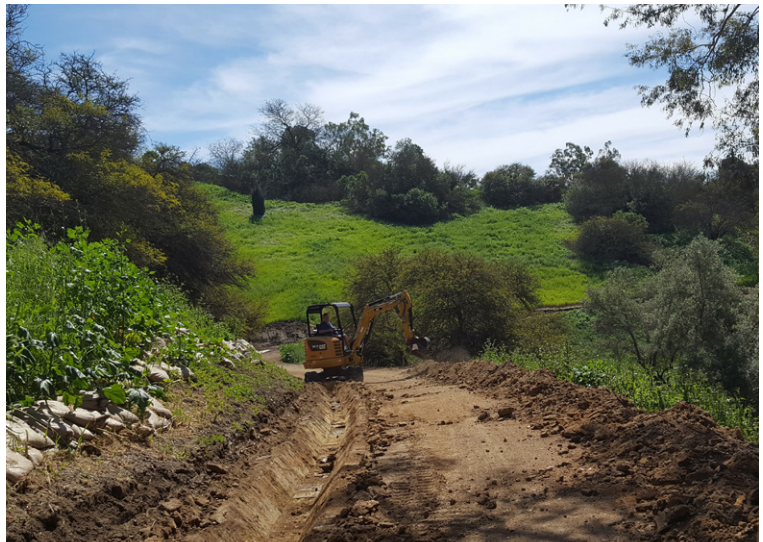
Creation of channel and anchor trench
