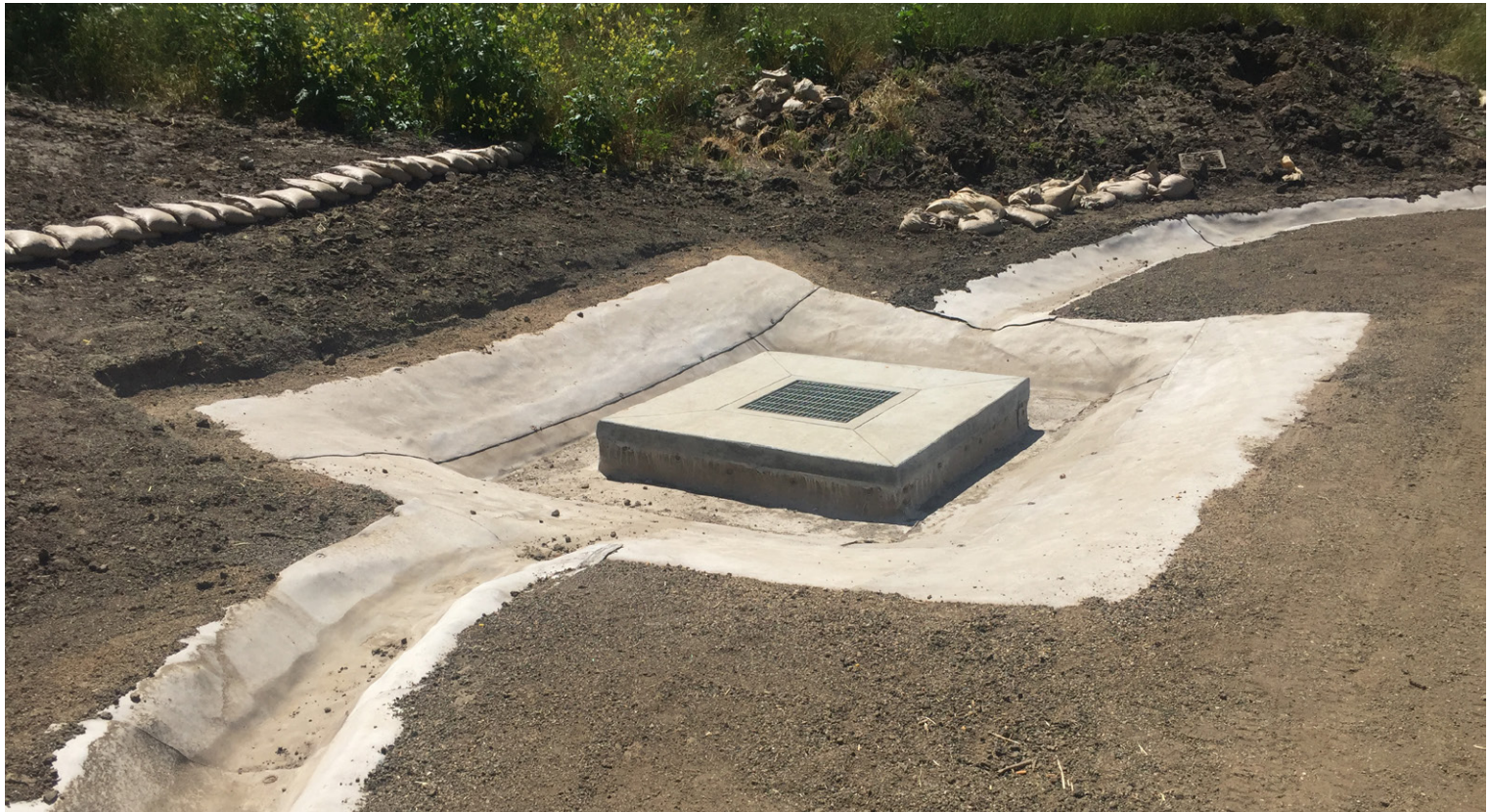
Completed channel and drainage section
