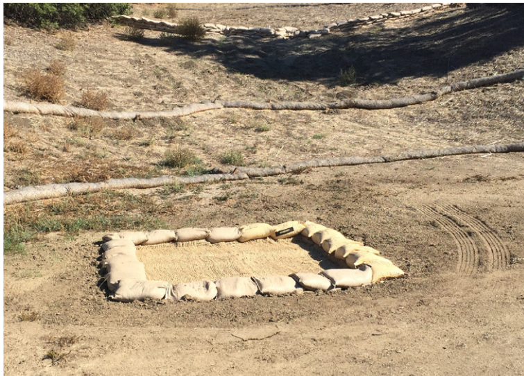
Drain prior to installation
