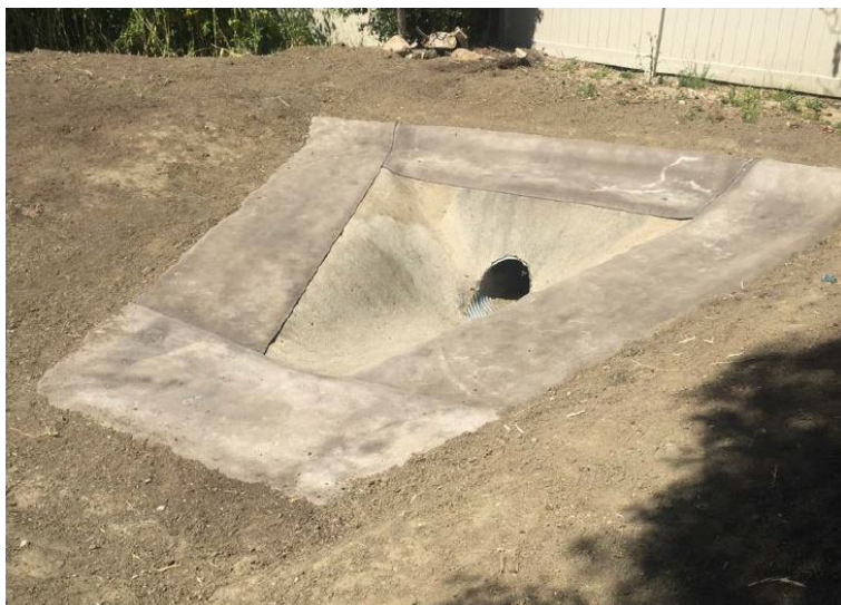
Completed drainage pipe section
