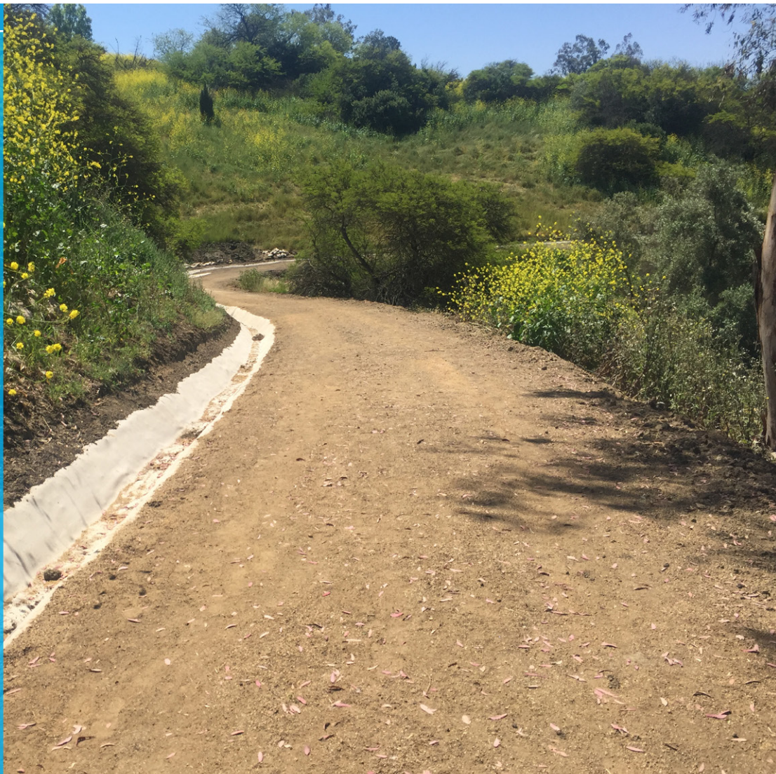
Completed channel along a stretch of the footpath
